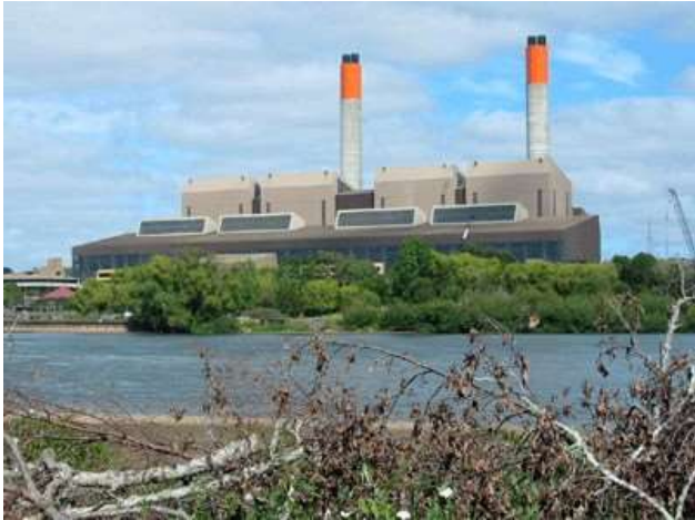
Fig 12 Huntly Power Station. Coal and gas fired
